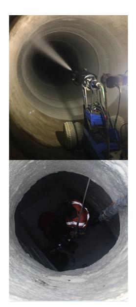
**360Ringtech® Robotics** flexibility allow for their use in pipe, vaults and other structures. The Orbital Spray Head can be mounted on a remotely controlled self-propelled crawler drone or on a skid mounted winch driven assembly.
